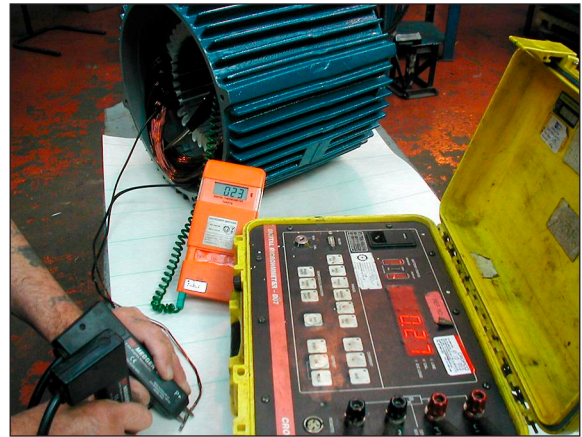
Figure 29. Measuring the resistance of a coil group. Note the meter leads are clamped securely to bare conductors; also note the ambient temperature thermometer.
